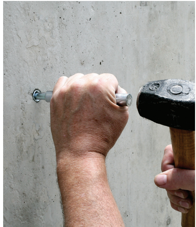
Anchor being set with hand setting tool.
