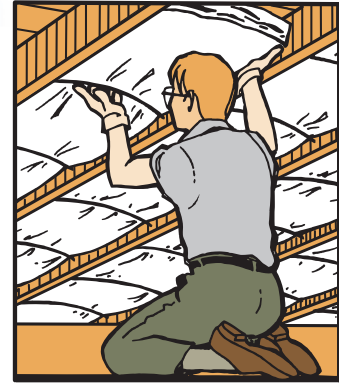
Typical IS Installation
