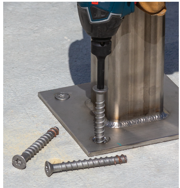
Titen HD Countersunk Installation
