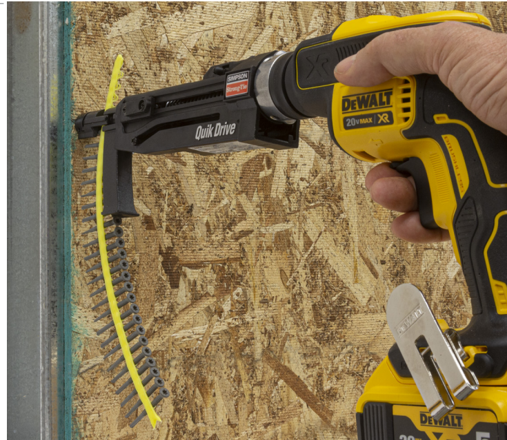
Quik Guard coated PPHD SHEATHING-TO-CFS screw installation using Quik Drive system
