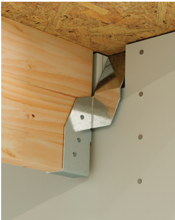
DGT fire wall hanger installation.
