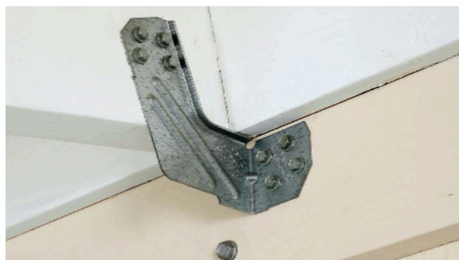
Typical HPTZ with SD10112 and SDS25112 installation.
